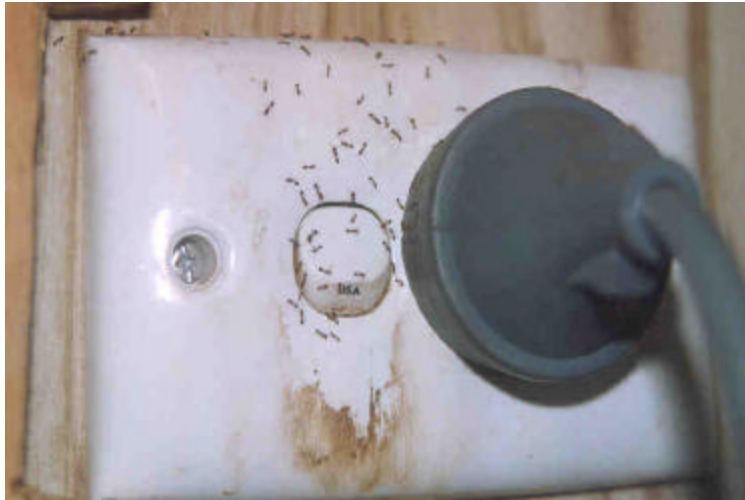
Singapore ant ( Monomorium destructor ) infested walls on Bathurst Island causing fire hazards. Photo courtesy of Ben Hoffman, Commonwealth Scientific & Industrial Research Organisation, Australia.
